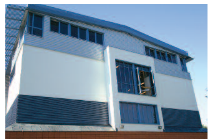
ERD louvre panels on the plant room, and Solarfin solar shading panels.
