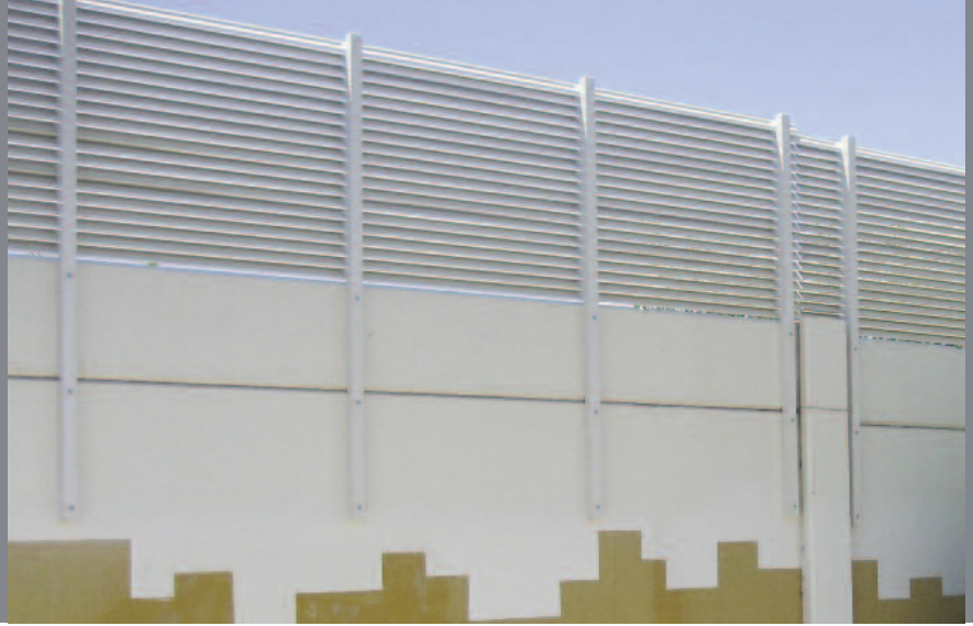
Roe Highway, Perth, Western Australia. 1UL/SH Louvre for screening.
