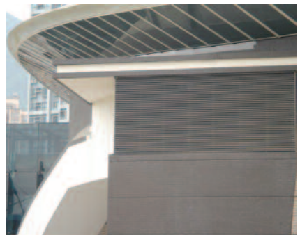
Universal Louvre for plant room ventilation and for controllable air inlet for the smoke extraction system.
